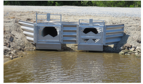
WATER CONTROL STRUCTURE
